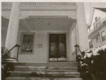
300 Norton Street, Yeshiva Gedolah, Original and Current Main Building
