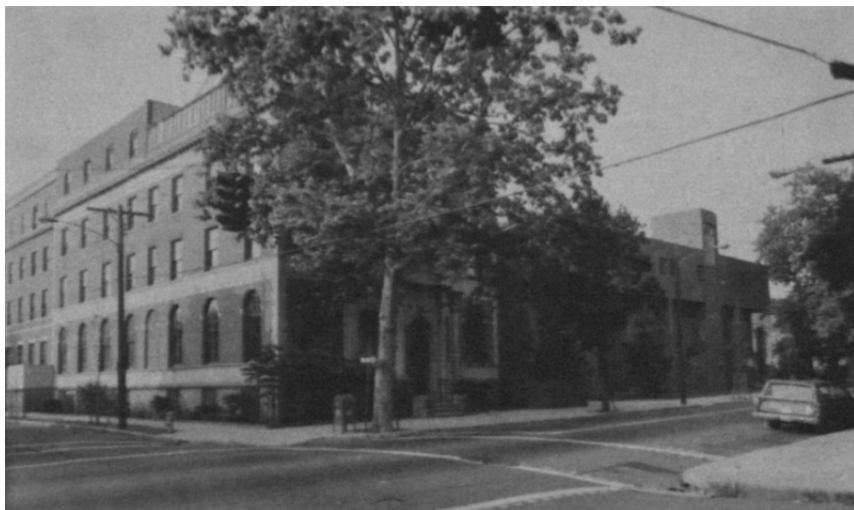
Figure 26: 169 Davenport Avenue with the 1976 addition
